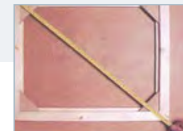
Check for distortion. Staple across corners for more stability.
