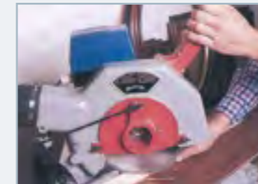
Mitre to required lengths allowing for expansion.
